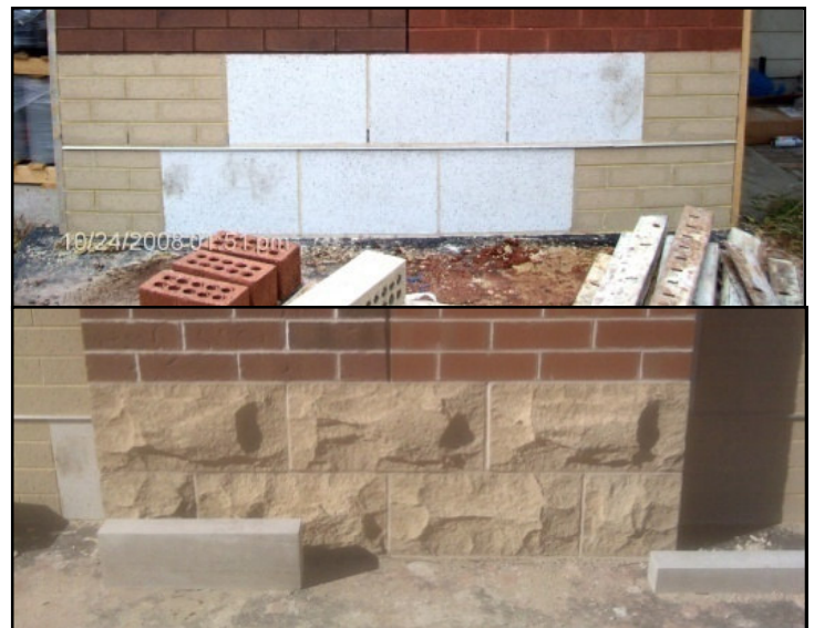
Figure 6 – Masonry Block Mock-Ups
