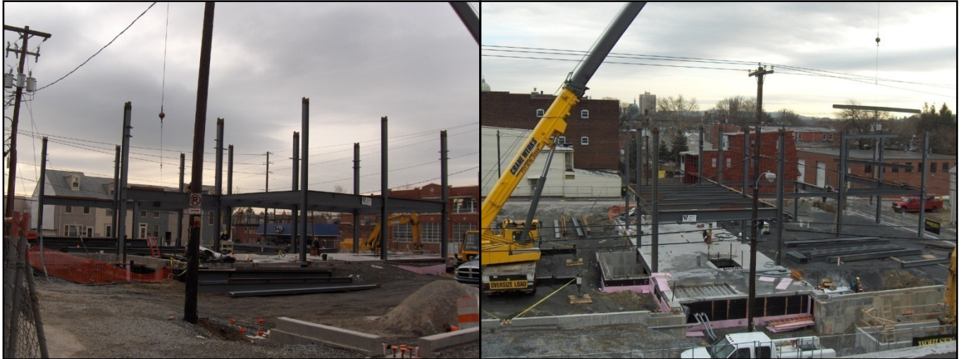
Figure 3 – Existing Utility Poles and Power Lines
